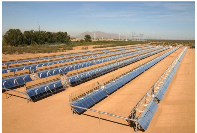
Fig. 1 The 10,300 m 2 solar plant began delivering 1 MW of electricity to the APS grid on December 27, 2005. The plant is currently operating without energy storage.
