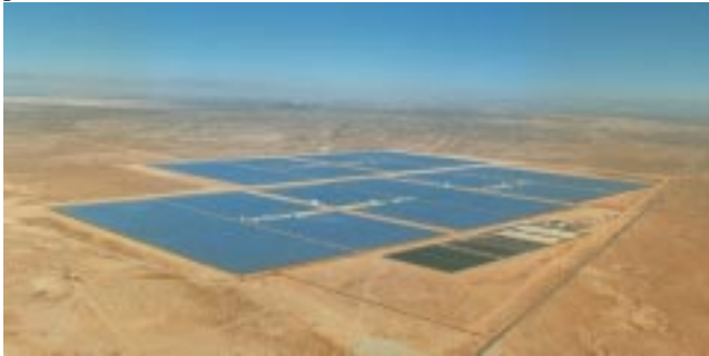
Figure 1. The 30MW SEGS III-VII parabolic trough plants in the California desert.
