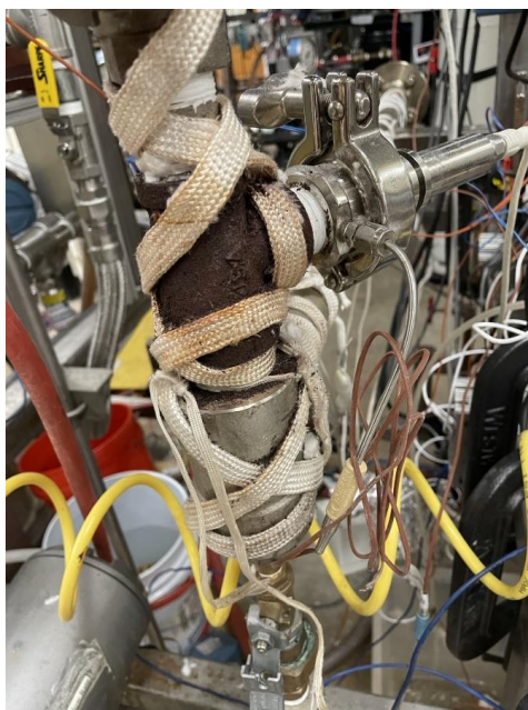
Figure G1: Rusted fitting that had a steam leak. The fitting was crumbling at the touch and an immediate replacement was needed.
