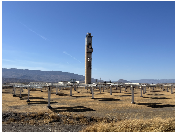
Figure 1.3: Power tower for receiver testing with a solar field in the foreground at Plataforma Solar de Almeria in Spain. Photo taken by author.
