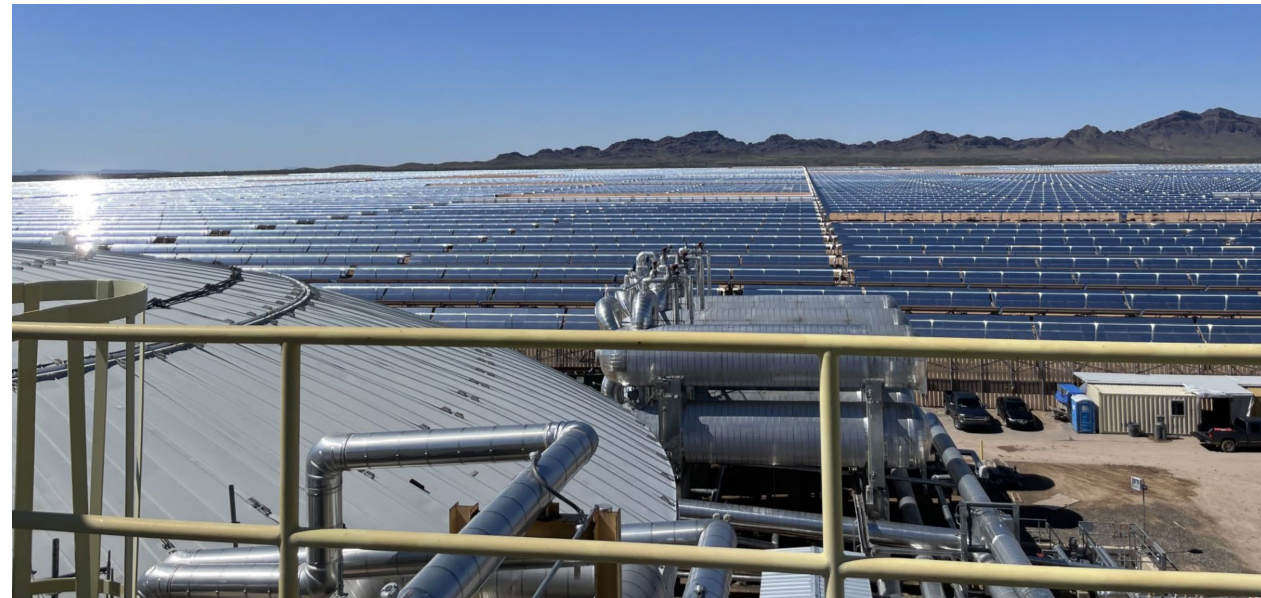
Troughs used at Solana
