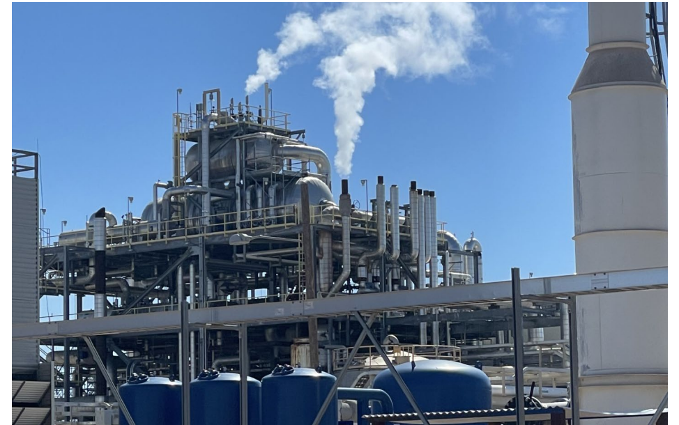
One of Solana's Power Blocks
