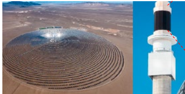
Heliostat field and tower receiver at Crescent Dunes CSP plant [1]
